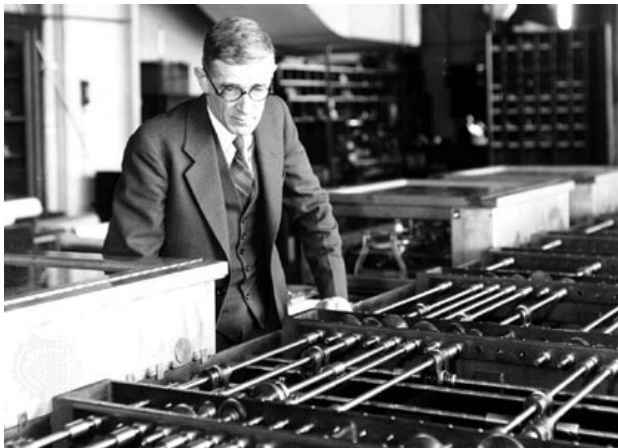
Differential Analyzer (Vannevar Bush, 1931) (solves Ordinary Differential Equations (ODE))
